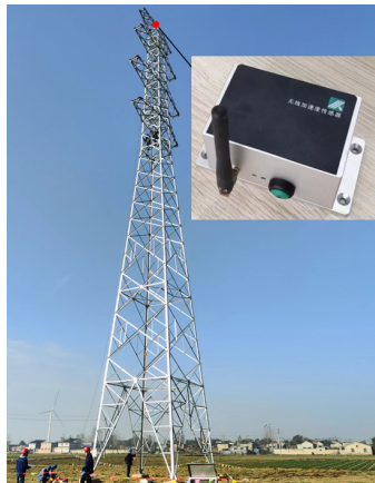
Fig. 2. Acceleration monitoring point location
