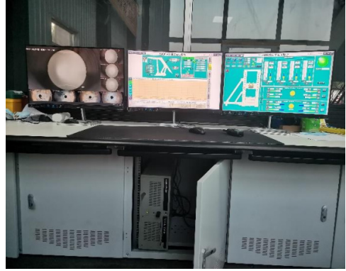
Fig. 11. Hydraulic support test bench console
