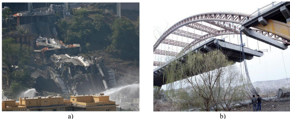
Fig. 1. Examples of bridge accidents: a) Morandi Bridge in Genoa, Italy, b) Kongquehe Bridge in Korla, China
