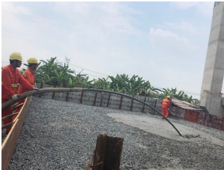
Fig. 2. Construction of a lightweight soil roadbed at the bridgehead
