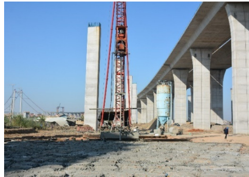
Fig. 3. Construction of cement mixing pile
