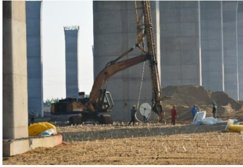
Fig. 1. Site view of the bridge
