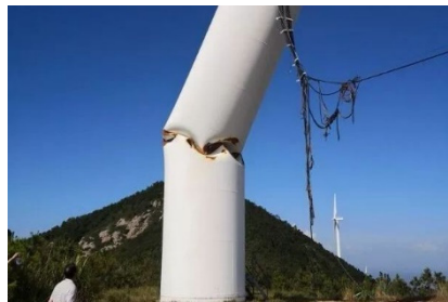
b) Damaged tower cylinder
