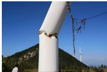
b) Damaged tower cylinder
