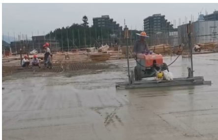
a) Concrete pouring with a laser paver
