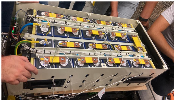
Fig. 14. Taking temperature measurements from the surfaces of the batteries
