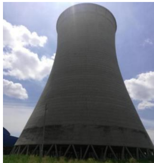
Fig. 3. Double curve cooling tower to be dismantled
