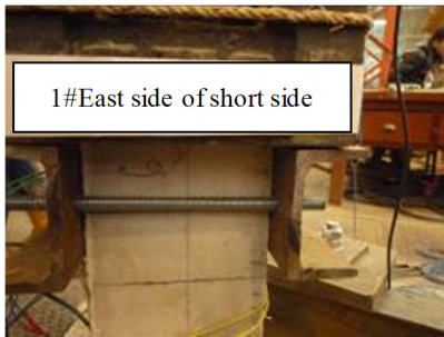
a) Status of the east side of the short side of pier 1#
