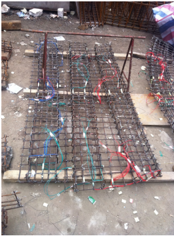
a) Steel binding
