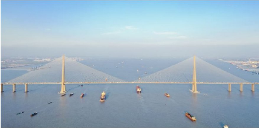
Fig. 1. Sutong cable-stayed Bridge
