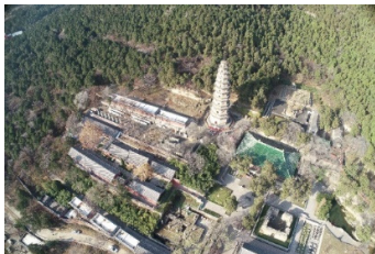
a) UAV oblique photography image
