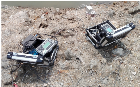
Fig. 5. Arrangement of blasting vibration meters
