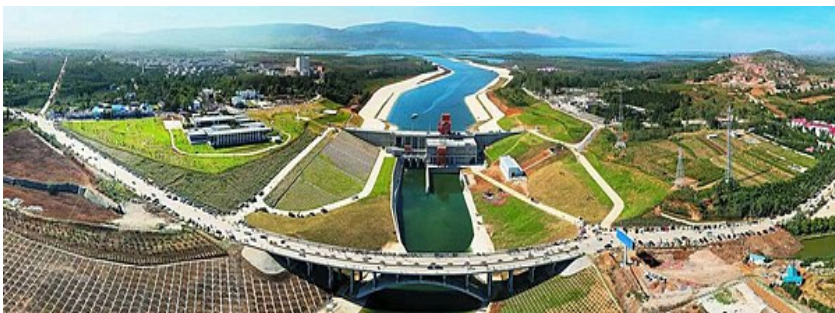
Fig. 6. Starting point of the central water channel in Sichuan
