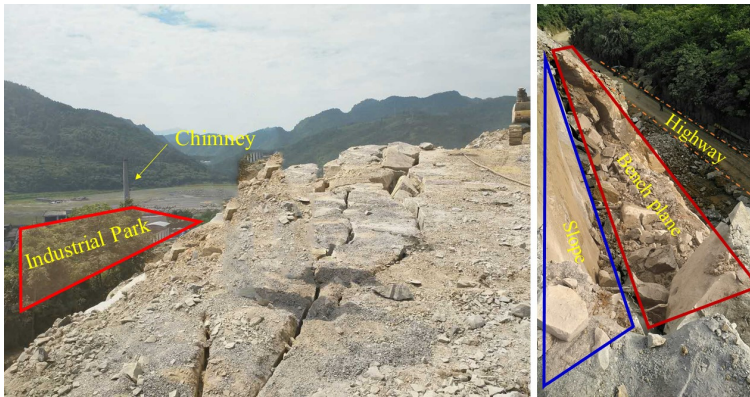
Fig. 1. Field test site of rock breaking
