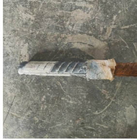
Fig. 12. Peeling failure of reinforcement and concrete
