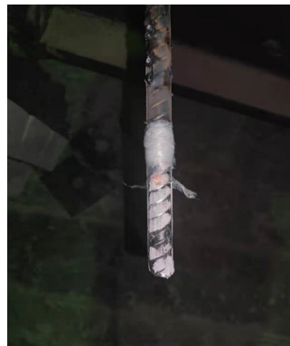
Fig. 4. Peeling failure of structural adhesive and reinforcement
