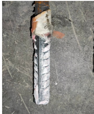
Fig. 7. Peeling failure of structural adhesive and reinforcement
