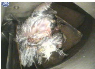
a) Bird stuck by the inlet guide vanes
