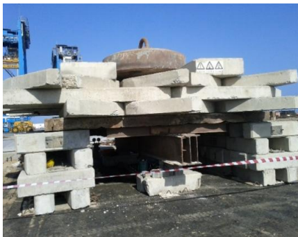
Fig. 2. Field plate loading test
