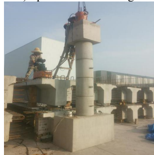
f) Prestressing tension operation
