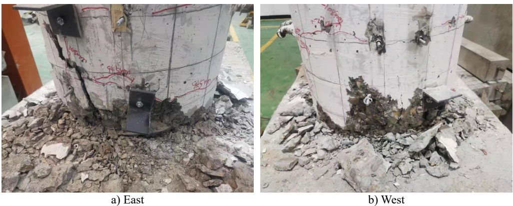
Fig. 9. The failure mode of MTSP2
