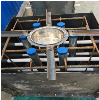
a) Preparation of mold for the segment 1 and load-end
