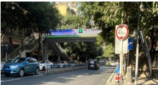
Fig. 5. Tested pedestrian overpass
