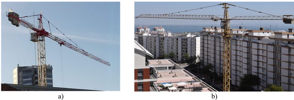
Fig. 2. Photographic register of both Tower Cranes: a) Arco do Cego (AC) and b) Alto do Olival (AO)
