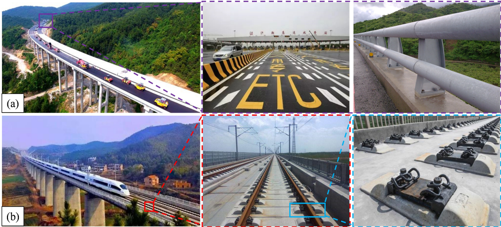
Fig. 1. Different bridge types: a) highway bridges; b) HSR bridges
