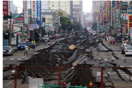
Fig. 4. An explosion occurred in a pipeline in Kaohsiung
