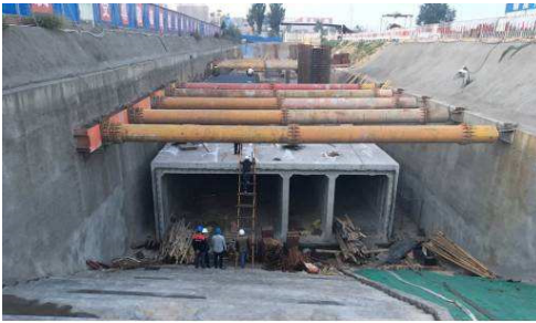
Fig. 1. An facility under construction in Beijing
