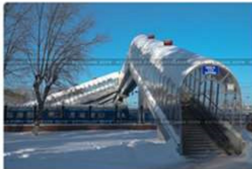
Fig. 3. The pedestrian bridge
