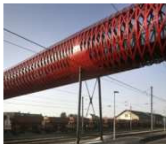
Fig. 1. Application of the proposed approach in railway transport systems (the pedestrian bridge)
