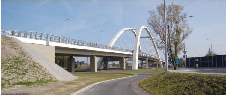
Fig. 1. A view of the viaduct
