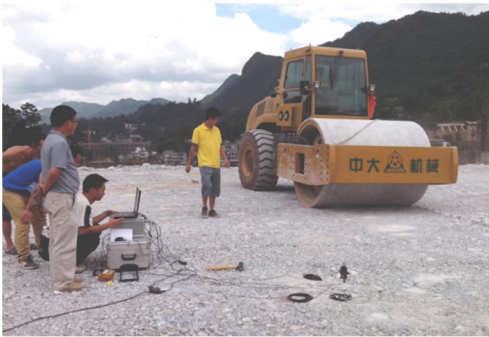
Fig. 2. Limestone subgrade field vibration test
