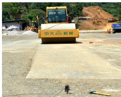
Fig. 4. Coarse-grained soil field vibration test
