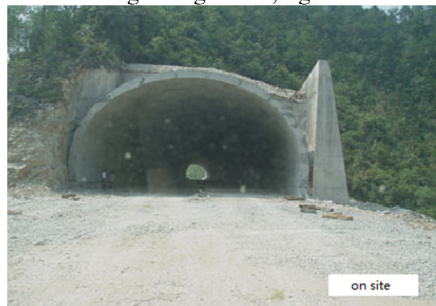
d) Zhuxia Section in the Huangshan tunnel, right line
