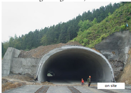
c) Zhuxia Section in the Huangshan tunnel, left line
