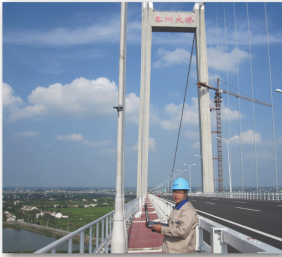
Load test and experimental modal analysis on most domestic bridges prior to commissioning
