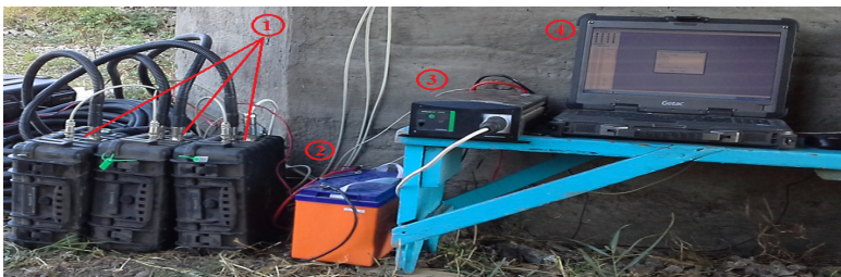
Fig. 3. General view of the mobile complex for strain gage measurement: 1 – measurement module, 2 – storage battery, 3 – sine inverter, 4 – A pilot computer
