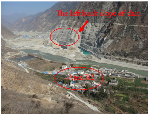
Fig. 5. Area B2 and surrounding blasting operation area
