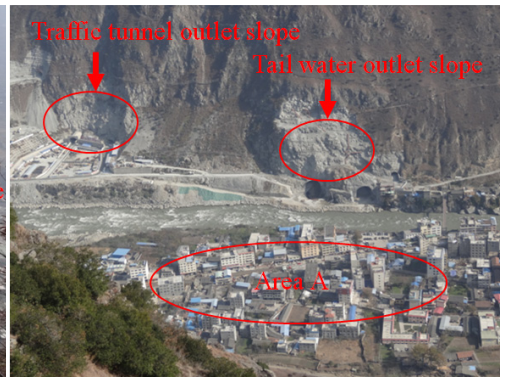
Fig. 4. Area A and surrounding blasting operation area
