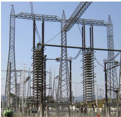
Fig. 1. Steel frame of converter station
