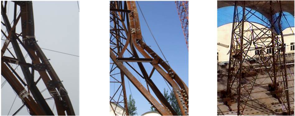
a) ±800 kV HVDC test tower b) 1000 kV HVAC test tower c) 500 kV HVAC test tower
