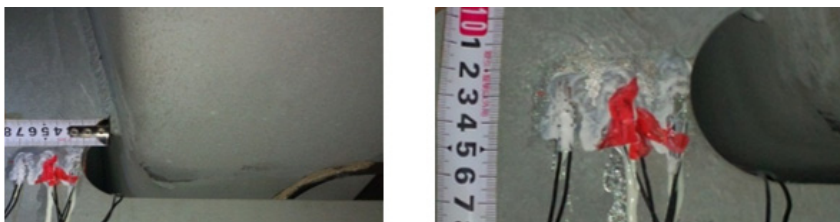
Fig. 6. On-site picture after adhesion of strain gauges
