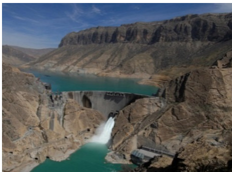
Fig. 2. General view of Karun IV dam
