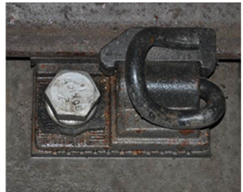
Fig. 2. The detail structural components of DZ III rail fastener
