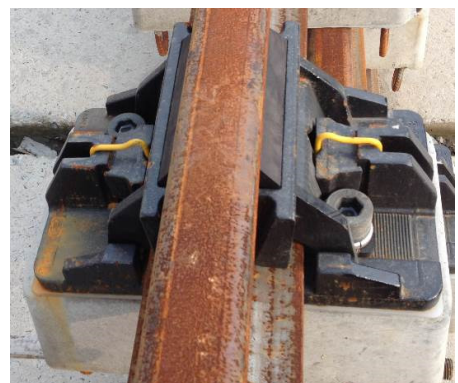
Fig. 3. The detail structural components of rail suspension fastener
