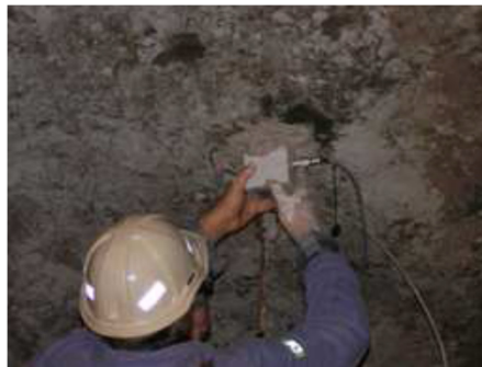
Fig. 2. The accelerometer located on the mining corridor roof
