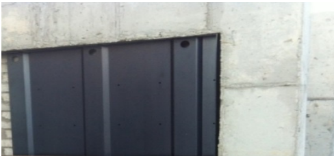
a) Installation waved panel
