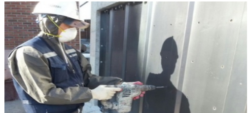
b) Drilling of holes in wall
