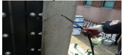
d) Application of epoxy
