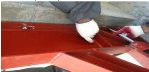
c) Injection of sealant
