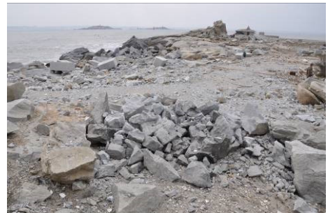
Fig. 14. The boulder after blast
