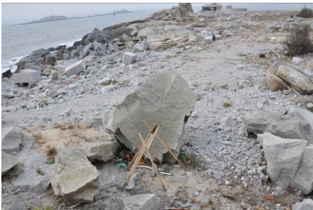
Fig. 13. The boulder before blast
