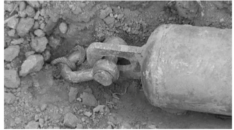
Fig. 15. The picture of the connection between pipeline and hinge ring
