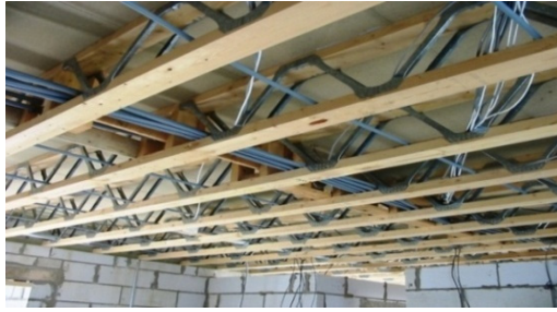
Fig. 1. Floor made of hybrid timber-metal beams
