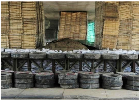
a) Flexible steel frame and sandbag walls
