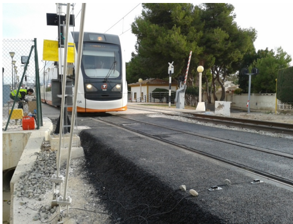
Fig. 8. Stretch of asphaltic track and accelerometers
