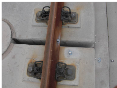
Fig. 4. Arrangement of in-situ acceleration sensors
