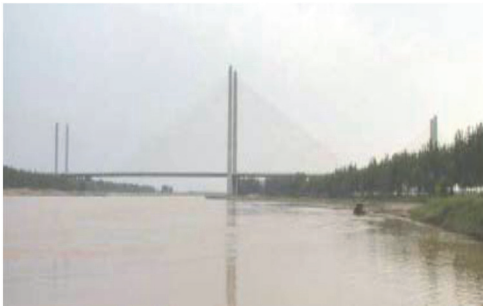
Fig. 5. Binzhou Yellow River bridge
