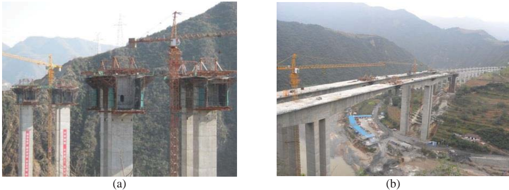
Fig. 5. Photos of a pre-stressed concrete Rigid Frame Bridge during different construction stage: (a) the zero block construction stage, (b) the closure up construction stage of the main span
