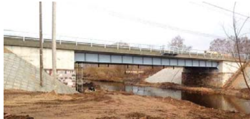
Fig. 2. General view of the bridge
