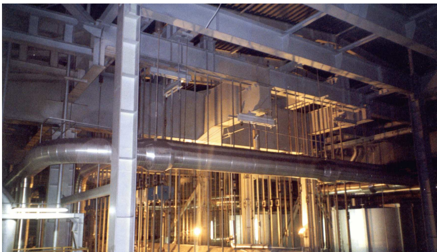
Fig. 1. View of combustion chamber's tension members
