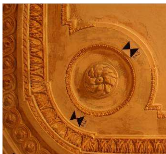
Fig 6. Orthophoto of the ceiling composed using points of triangulation
