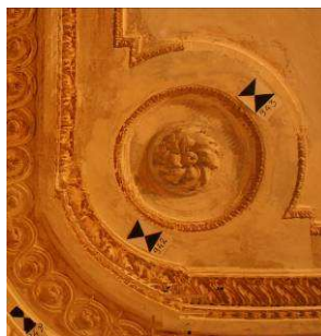
Fig 7. Orthophoto of the ceiling composed using points of triangulation and structural lines data
